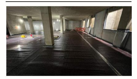
Internally, we are working in the basement with blockwork and waterproofing. We plan to start internal fit-out to our flats as soon as the roofing is in place.
